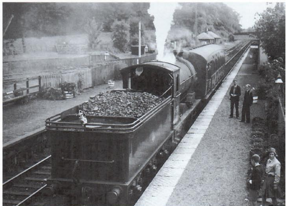
J37 No.64598 pauses at Buchlyvie before taking the Aberfoyle branch at Buchlyvie Junction with the local passenger shuttle from Blanefield on 18th September 1951. The line between Lennoxtown and Aberfoyle was closed to passenger traffic just two weeks later, from 1st October 1951. (G. H. Robin)
