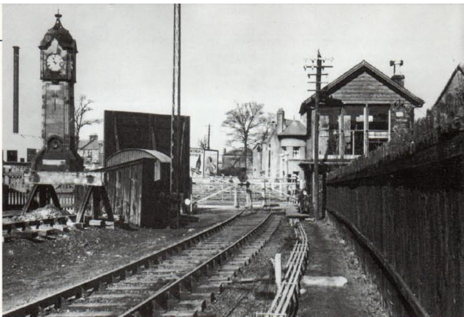
Stirling New Bridge signal box controlled a busy level crossing on the main Stirling to Bridge of Allan road. Single line tablet working ended there and block working applied on the double track section on to Stirling North box and the station. The site is now a busy traffic roundabout, with the ornamental Bridge Clock Tower, presented to the town by Provost David Bayne in 1910, marooned in the centre of it. (Author's Collection)
